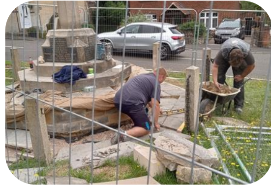
14/08/2024 - Contractors levelling the ground using a spirit level.
