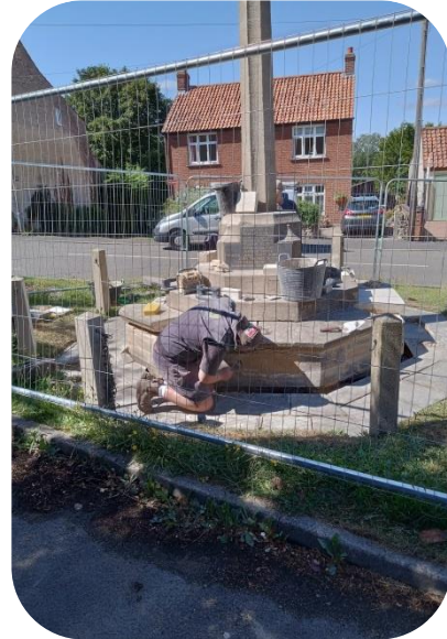
16/08/2024 - New bricks and old bricks being set and pointed
