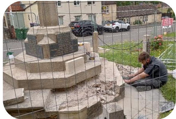
25/07/2024 - A contractor continuing to carefully scraping out old pointing.
