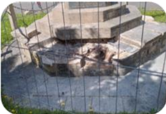
23/07/2024 - The old stones have been cleaned in readiness for the new stones to be put in place.
