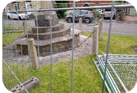
14/06/2024 - The work has to be done by hand tools only.
