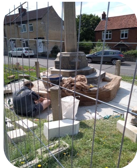
29/07/2024 - New stones are laid on the grass ready for carefully being placed onto the War Memorial.
