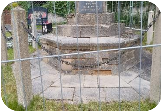
14/06/2024 - Work starts on scraping out the old mortar.
