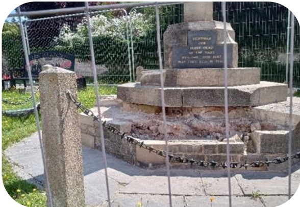
23/07/2024 - The loose mortar and old stones have been removed.
