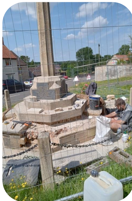
31/07/2024 - Contractor working in the hot sun preparing the area for re-pointing.
