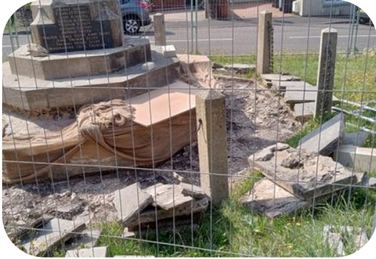
12/08/2024 - Preparation for replacing the bottom slabs.
