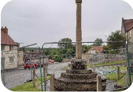
13/06/2024 - Fencing is erected around the War Memorial
