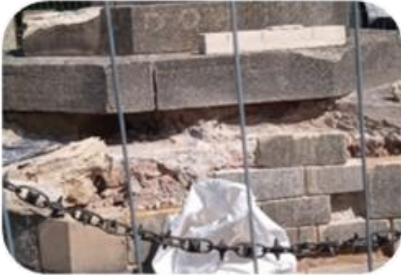
18/07/2024 - Work continues on removing the old pointing and concrete.
