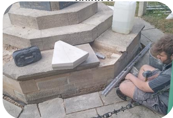
16/08/2024 - New bricks and old bricks being set and pointed
