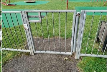
**Action:** Take corrective action to ensure that the gate closes in 4-8 seconds
