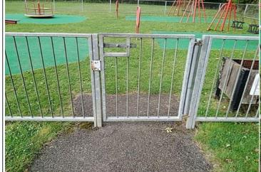
**Finding:** The gate is closing too quickly (less than 4 seconds)
