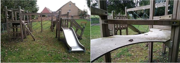
**Finding:** The item fails to meet the requirements of BS EN **Action:** Refer to the manufacturers for advice. 1176 Part 1 4.2.7.2 for head and neck entrapment where the opening between the lowest balance beam and the grey platform below is less than 230mm.
