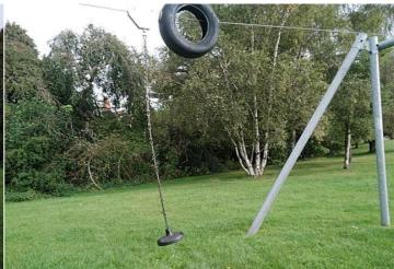
**Finding:** The seat is less than 2.0 metres from the post when extended at 45 degrees at the end of the area of travel minimum distance is maintained and does not meet the requirements of BS EN 1176 Part 4
