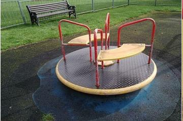
Finding: Slight vertical movement in the platform may be due to wear in the bearings.
