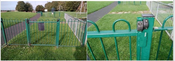
**Finding:** There are openings that are less than 12mm that could trap or crush fingers
