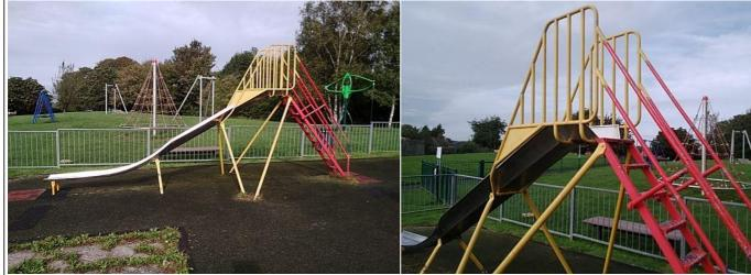
**Finding:** The item fails to meet the requirements of BS EN Action: Monitor - No remedial work recommended 1176 Part 1 4.2.7.2 head and neck entrapment in the barriers and/or steps
