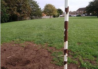
Finding: Corrosion Action: Rub down and repaint as required
