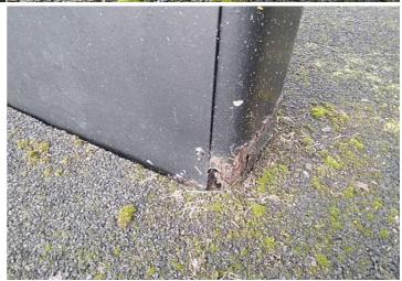
**Finding:** Parts of the steel on this item have corroded excessively and the metal has perforated in places at the base of the main stanchion
