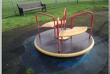
**Finding:** The safety surface under or around this unit has been damaged
