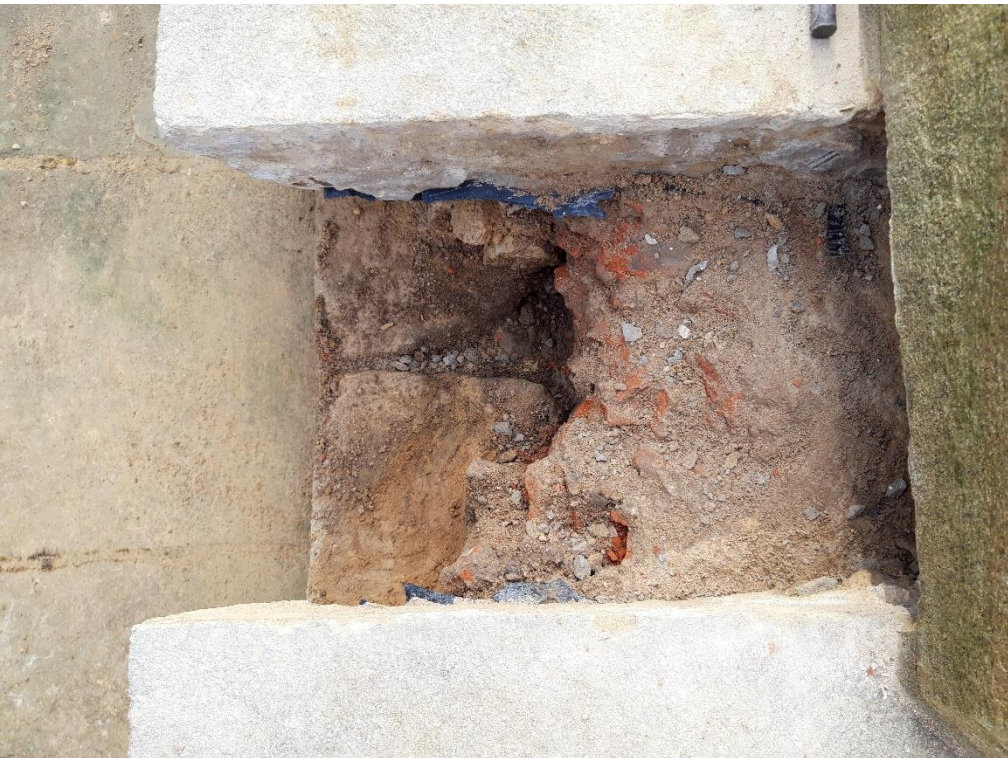
Rubble core and outer stonework
