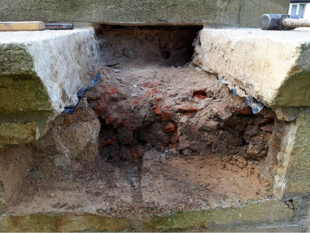
Rough bound rubble core
