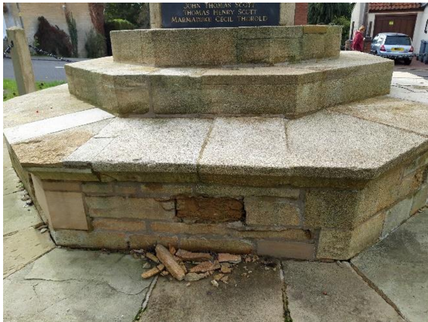
Fig. 3: The East plinth elevation before the investigative section.
