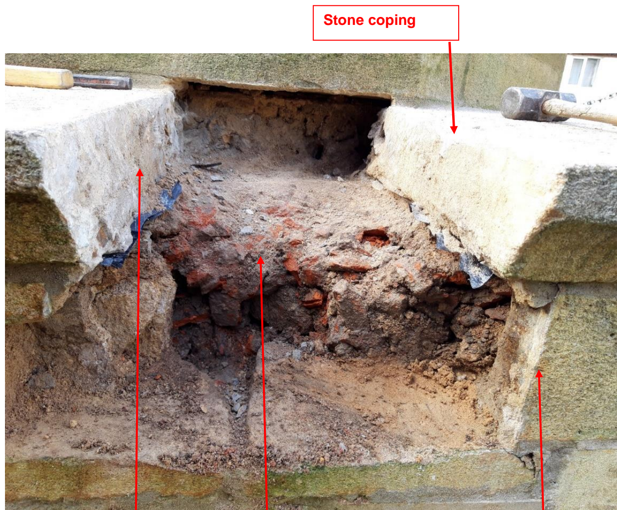
Fig. 4: Picture of the War Memorial structure after the investigative section.
