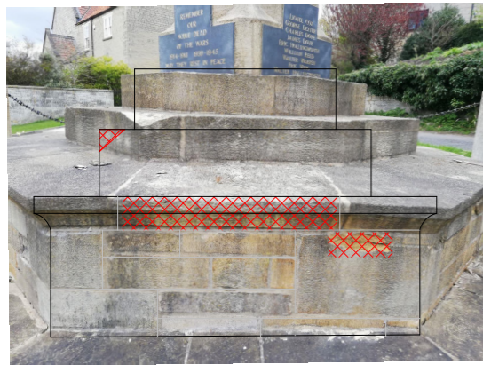
Side H (Southwest)
