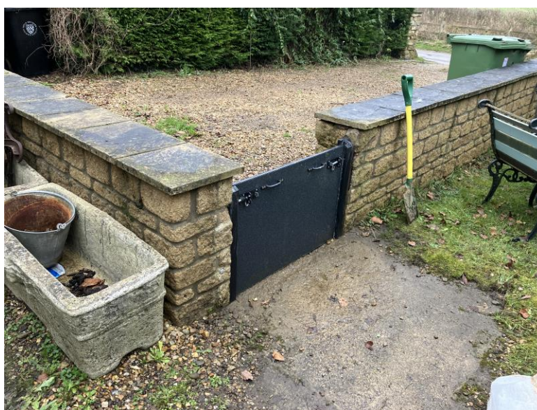
Figure 14: The demountable defence outside Pheasant Cottage that has replaced the steps as built in the original design. Provided by Environment Agency.
