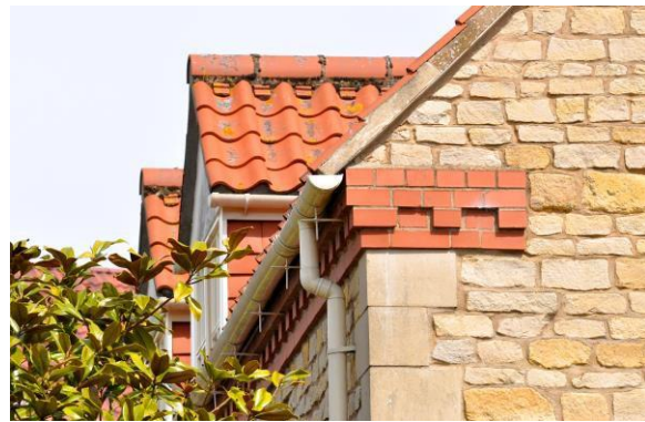
Gabled dormers and red brick oversailing courses with coursed limestone rubble walling .
