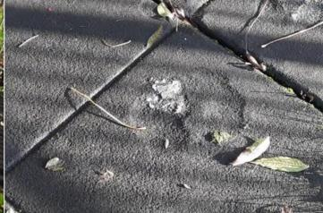
Finding: There is fire damage to the surfacing
