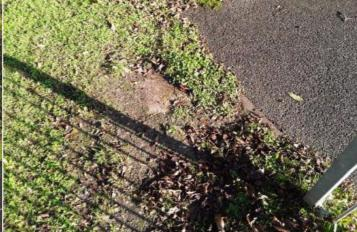
**Finding:** The surface has eroded around the entry points and may be slippery in wet conditions
