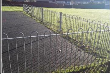
**Finding:** There is / are post caps missing or damaged on the fence
