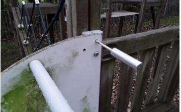
Finding: There is/are finger entrapment/s adjacent to the slide entry and the item fails to meet the requirements of BS EN 1176 Part 1 4.2.7.6 Entrapment of fingers
