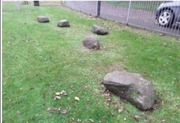
**Finding:** The fence forms a hard object within the falling space of the boulders in contravention of the requirements of BS EN 1176 Part 1
