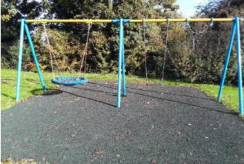
**Finding:** One seat has been removed and the chains wrapped to isolate from use however the area is still accessible and the means of isolation has either introduced additional hazards that may cause harm in the event of users accessing the area or is insufficient to stop users from accessing the chains
