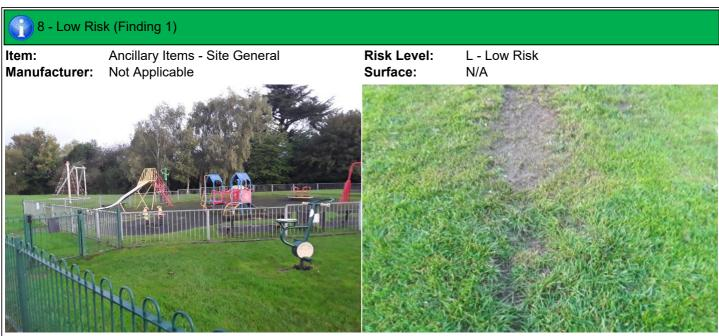
**Finding:** The grass mats are silted up, the soil is compacted **Action:** Reinstate as required and the area will become very slippery when the soil is wet.
