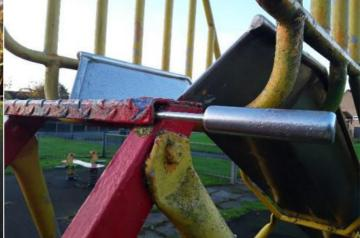
Finding: There is/are finger entrapment/s in the structure and the item fails to meet the requirements of BS EN 1176 Part 1 4.2.7.6 Entrapment of fingers
