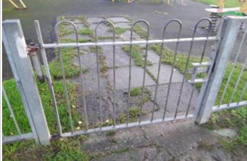
**Finding:** The concrete base under the gate is uneven creating trip hazards
