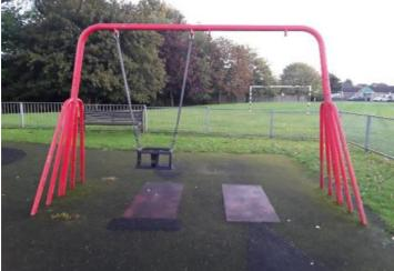
**Finding:** The seat clearance from finished surface level to the underside of the seat is too low and does not meet the requirements of BS EN 1176 Part 2 (350mm minimum clearance required)
