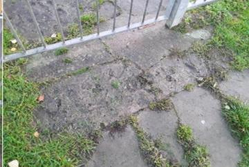
**Action:** Repair the damaged areas of concrete to provide a uniform surface
