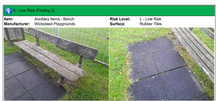
**Finding:** There are gaps opening in between the tiles in front of the bench
