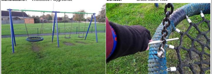
**Finding:** The chain openings are in excess of the 8.6mm as **Action:** Monitor - No remedial work recommended recommended by BS EN 1176
